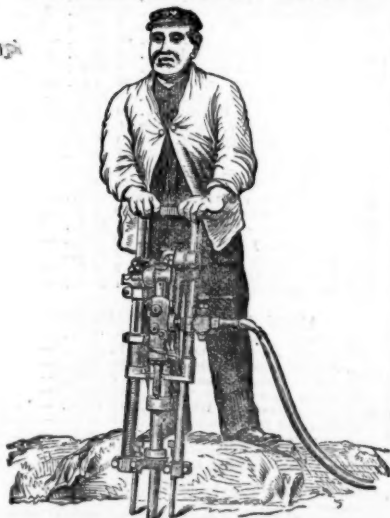
ARRANGEMENT FOR SHAFT SINKING AND QUARRYING.
